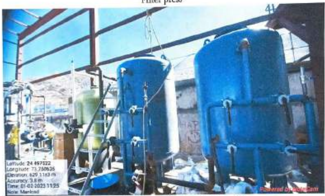
Pressure Sand Filter and Activated Carbon Filter
